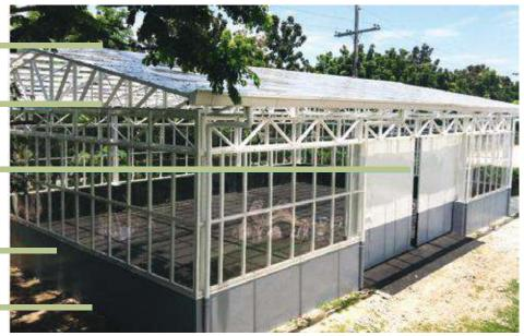
The solar sludge-drying facility uses zero electricity for drying and exhaust.
