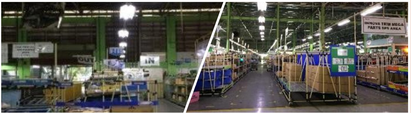
Aligning of light fixtures to properly illuminate Team Members' work areas
