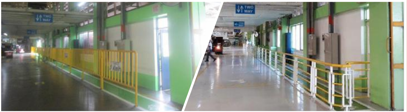
Re-painting of floor guides and markers to clearly establish areas for pedestrians and moving vehicles
